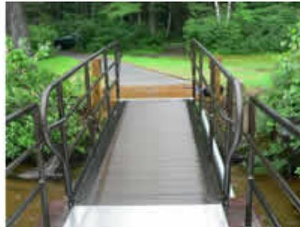
ADA style ramp w/anodized aluminum deck
